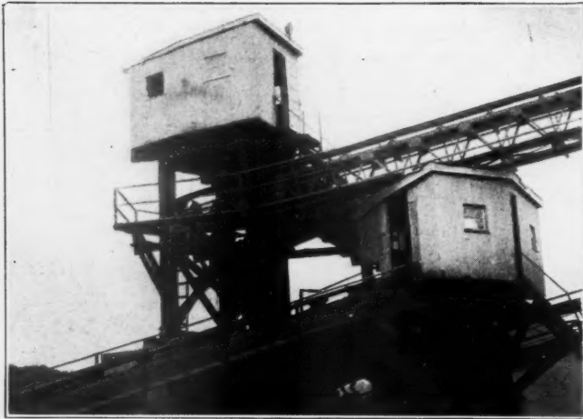
Gravel Comes up Conveyor in Foreground Feeding Through Washer to Lower Horizontal Conveyor. Sand Goes on Upper Conveyor
